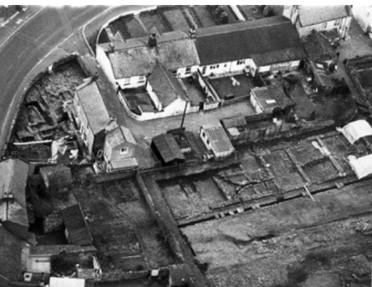
Courtyard building during excavation (DCC)
