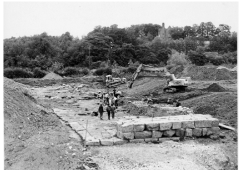
Bridge foundations being uncovered in 1972 (DCC)
