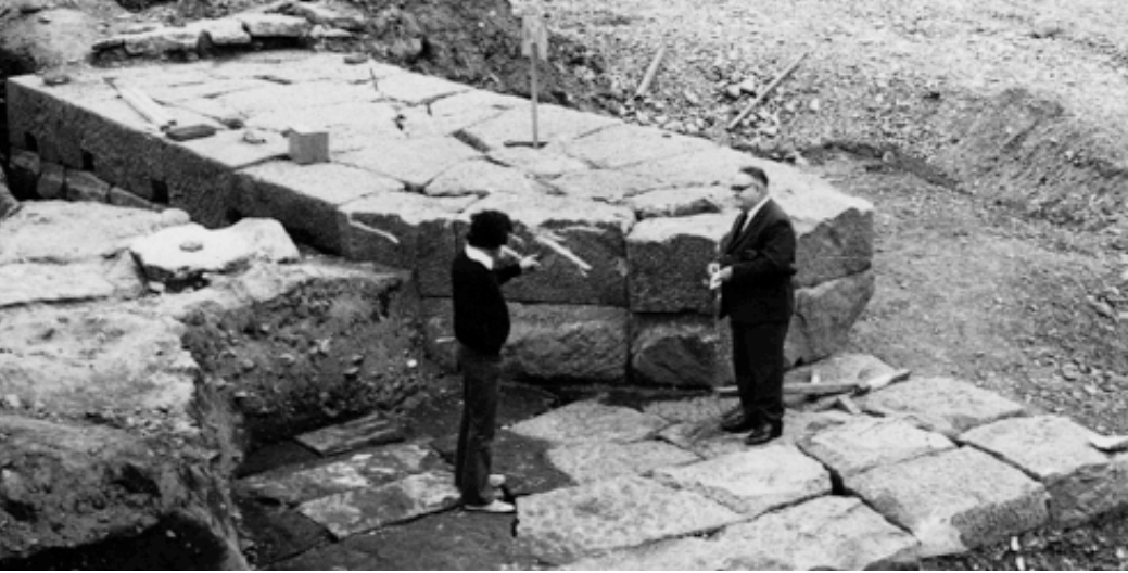
South bridge abutment during excavation (DCC)
