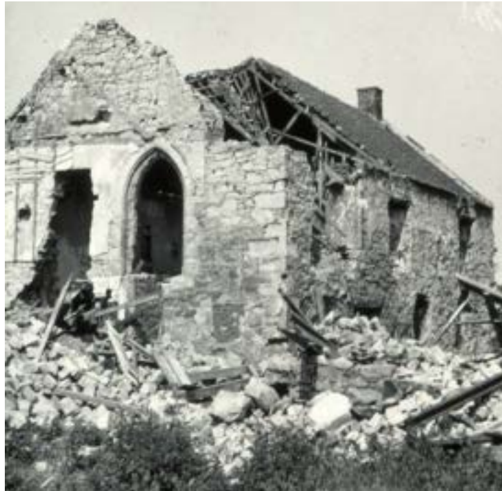
Figure 33: The farmhouse from the south-west during demolition in the early 1960s
