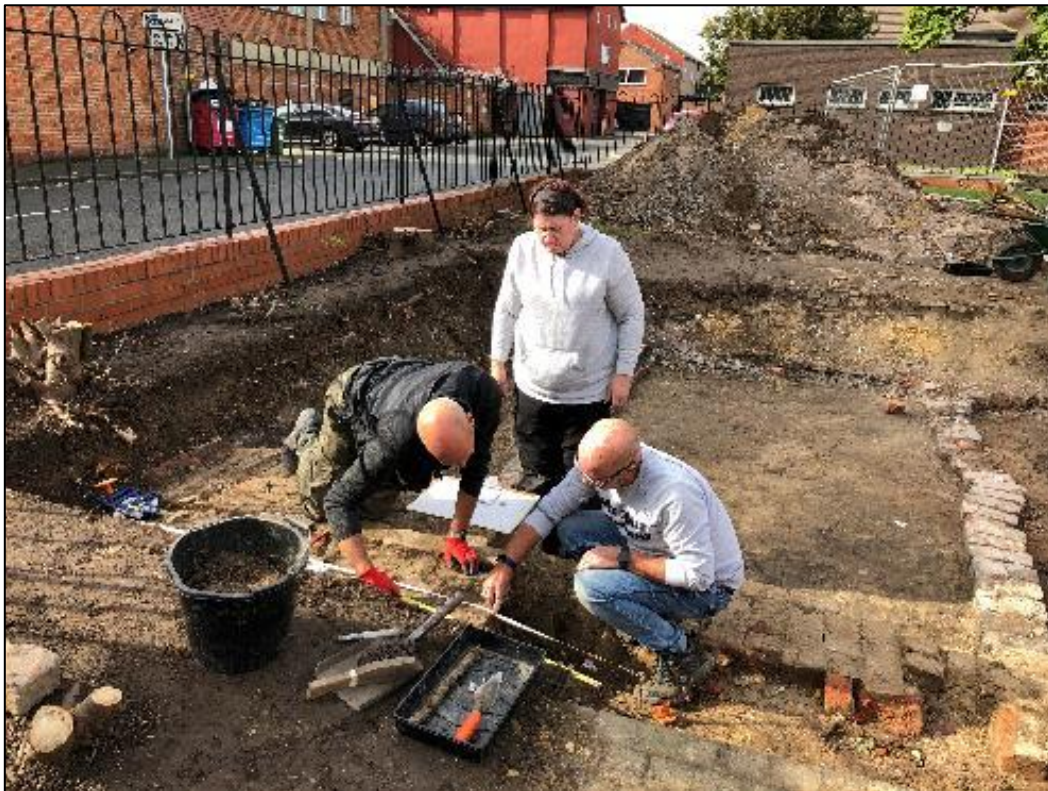
Figure 26: Planning the foundations
