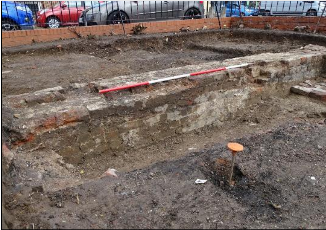
Figure 17: North wall foundation (8) south facing elevation
