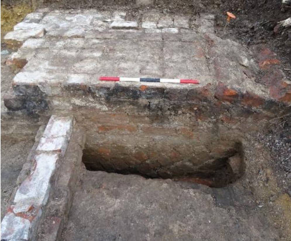
Figure 19: Inverted arch foundation (9) exposed in section, looking east
