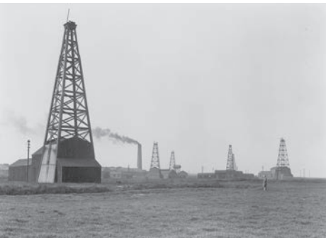
Drilling Rig near Greatham (IH)
