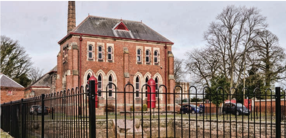
Tees Cottage Pumping Station (PG)
