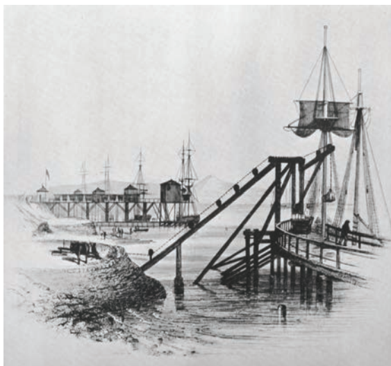
Clarence Railway coal staithes
