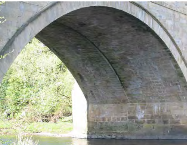
The underside of the arch and the join (left, upstream) of the single carriageway medieval bridge and the later, widened 18th century bridge, Piercebridge
