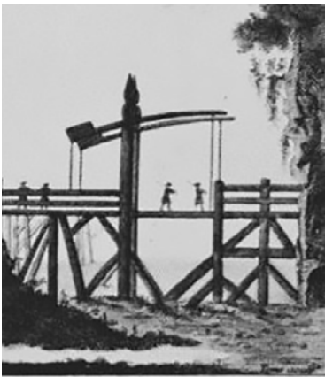
Wooden drawbridge, Clifford's Tower, York, late 17th century.
