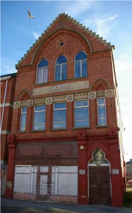
Fig 24: Clephan North End Engineering Works, 54-56 Norton Road
