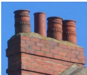
Fig 22: Chimney pots, 22 Dovecot Street.
