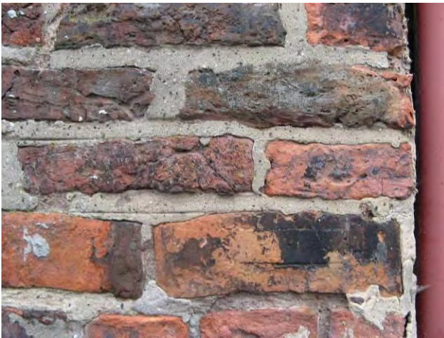
Fig 6: The top bricks are 18 th century and the bottom ones are 19 th century patching.
