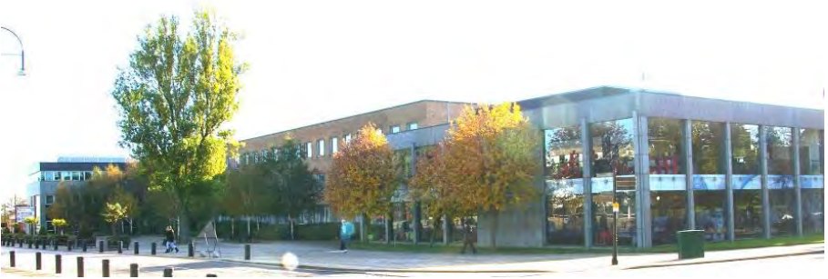
Fig 44: Stockton Library and Municipal Buildings
