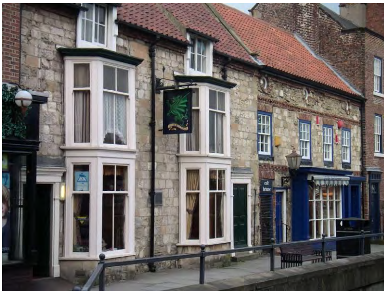
Fig 5: 17 th century stone buildings, Finkle Street – some of the stone may have come from the castle
