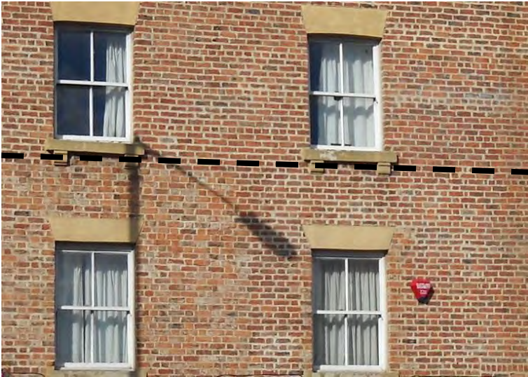
Fig 10: Number 153 High Street details of windows and bonding – line shows change in brick bond where building was increased in height
