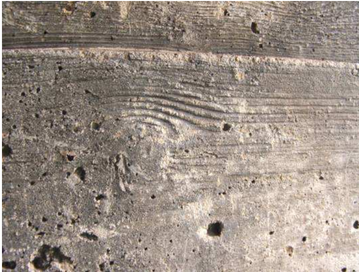
Imprints from wooden plank (top) and corrugated iron shuttering (below)
