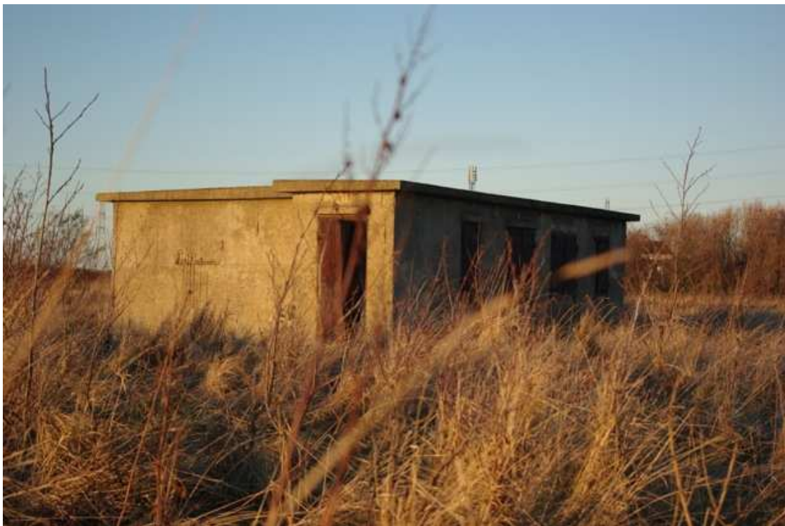
Surviving ammunition store at former Saltholme battery
