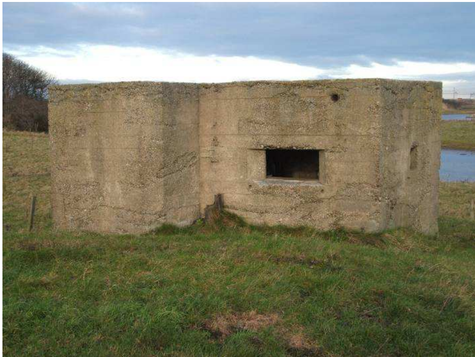
Pillbox built into an unfinished railway embankment at Greatham Creek
