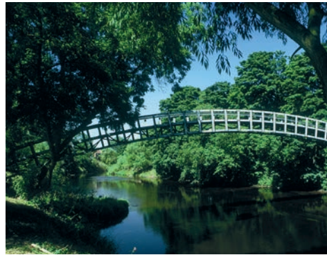
Fishlocks Bridge (RG)
