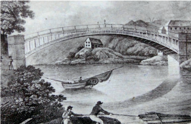
Yarm Iron Bridge (AB)
