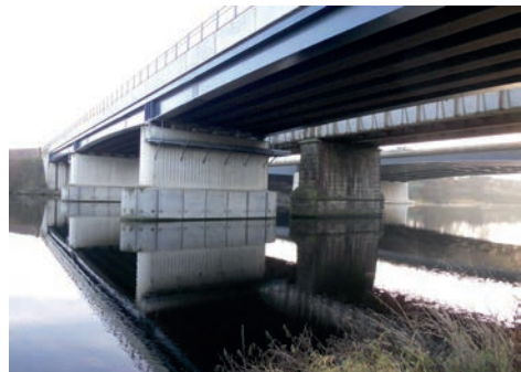
New Rail Bridge with 1906 bridge on 1844 stone piers and Surtees bridge behind (AB)
