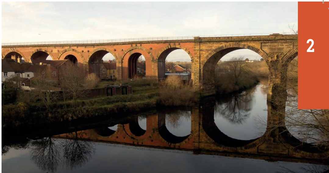
Yarm Railway Viaduct (AB)
