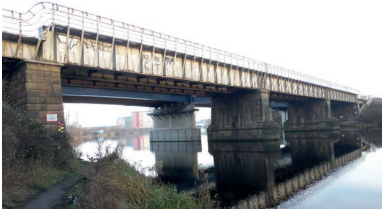
1906 bridge on 1844 stone piers (AB)
