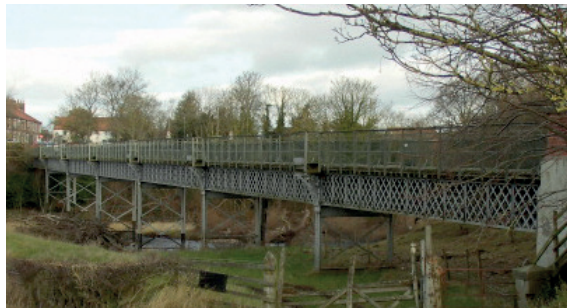
Low Hail Bridge (AB)
