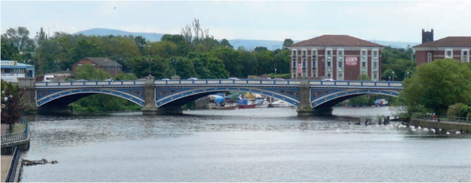
Victoria Bridge (AB)
