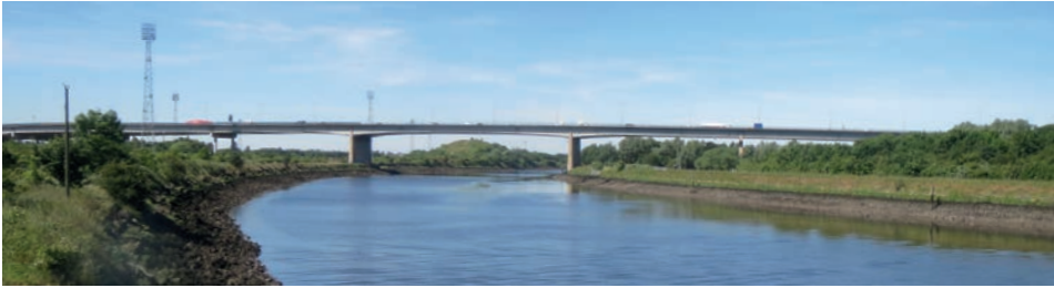
A19 Tees Viaduct (AB)
