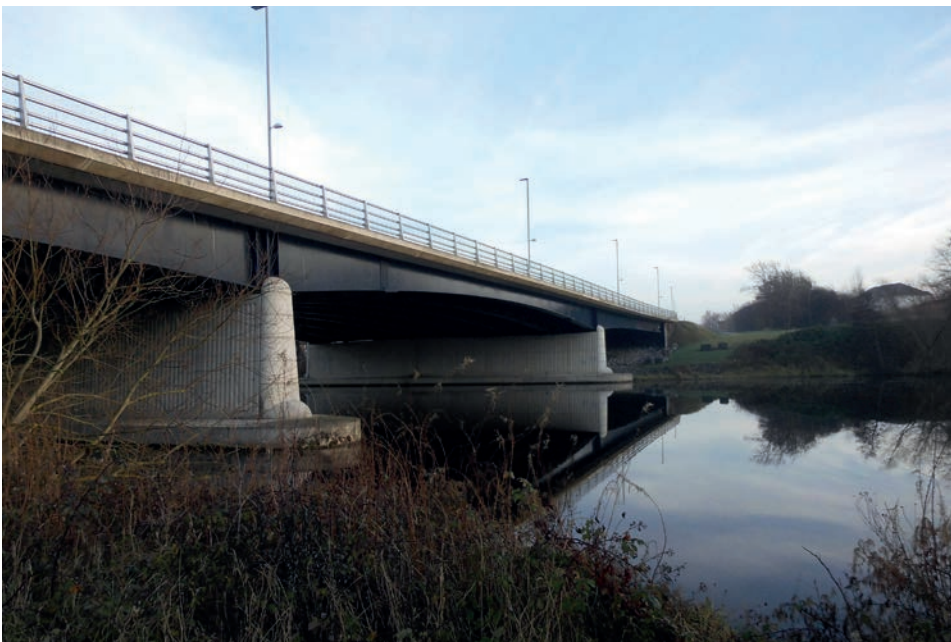
Surtees Bridge (AB)
