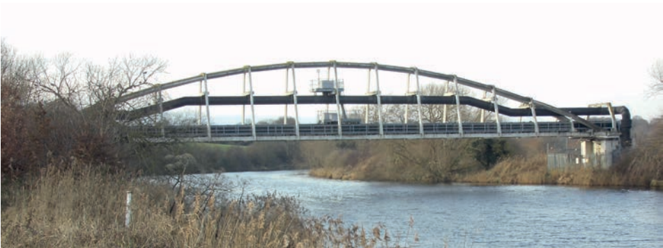
Preston Pipe Bridge (AB)
