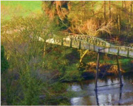
Girsby Bridge (AB)
