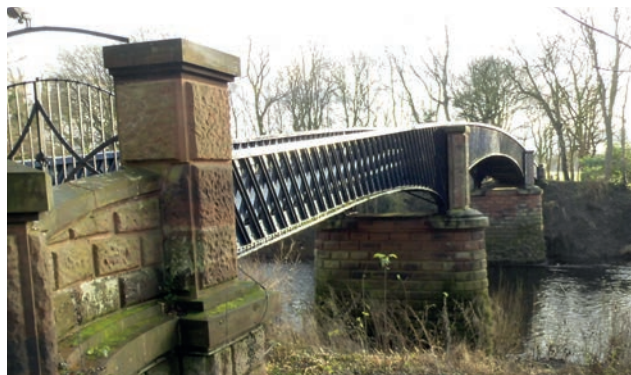
Neasham Hall Bridge (AB)
