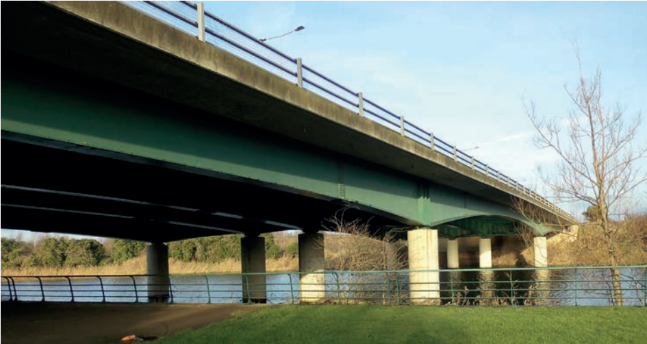
Jubilee Bridge (AB)
