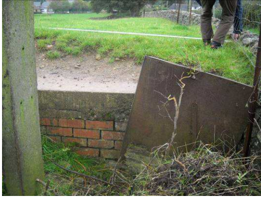
Figure 20 Air Raid Shelter, North Hart Farm, showing door and concrete roof
