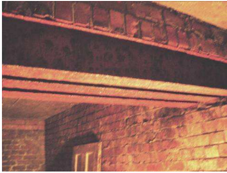
Figure 24: Air Raid Shelter Manor Croft, Hart, Roof with Steel Reinforcing Beams
