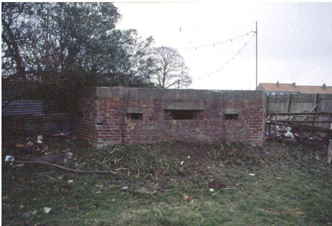
Figure 3: Demolished Pillbox to the rear of the Raby Arms (Tees Archaeology Archive)
