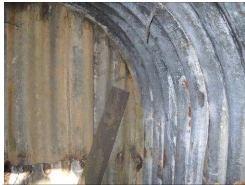
Figure 19: Interior of Anderson Shelter, Hart Station
