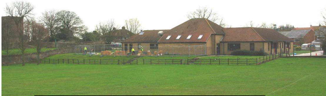
Figure 14: View of site of former military and POW camp
