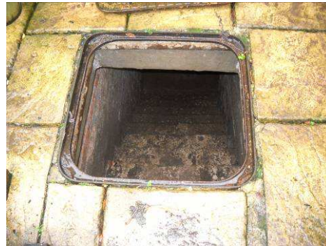
Figure 23: Air Raid Shelter Manor Croft, Hart, Entrance
