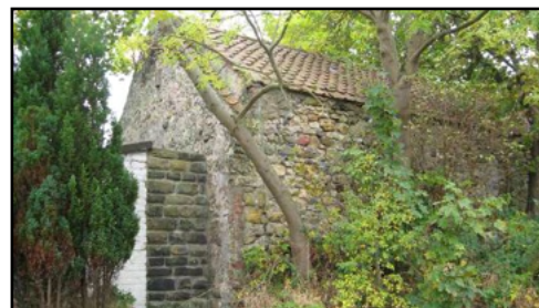
Plate 2. – 19 th century Outbuilding behind Beckwood House
