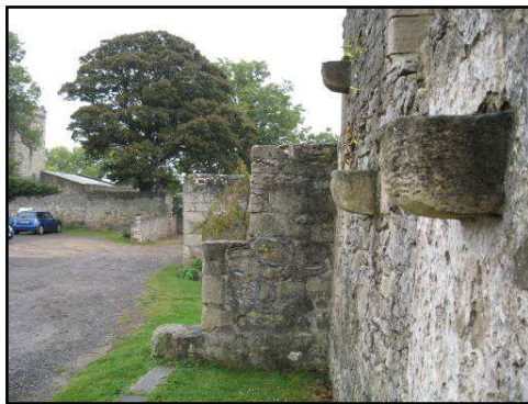
Plate 44. – Detail of joists in Brus Wall
