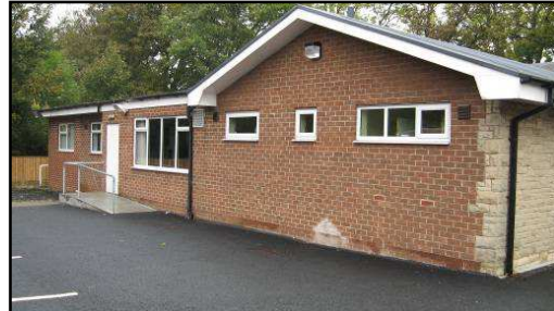
Plate 30. – Hart Village Hall, on the corner of Front Street and Butts Lane
