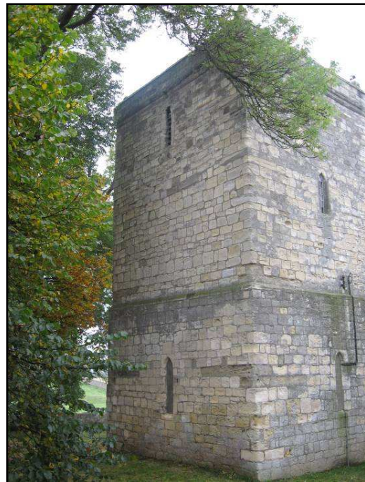
Plate 53. – St. Mary Magdalene Church exterior, showing the south east corner of the Tower. Note the two large, darker stone slabs dressing the corners at intervals.
