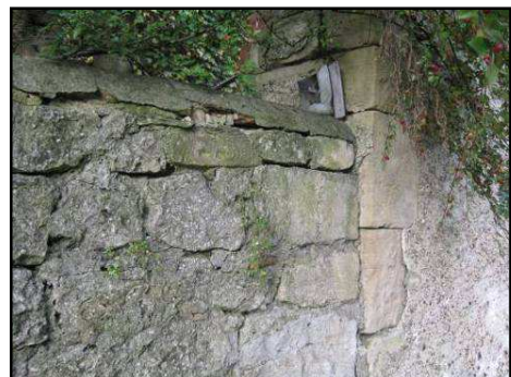
Plate 48. – Detail of join between Wall 5 & 6
