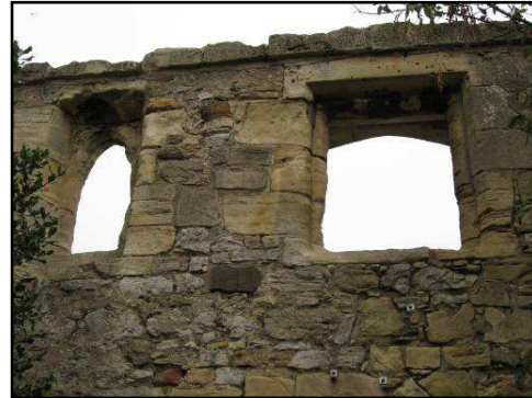
Plate 43. – Two windows in Brus Wall
