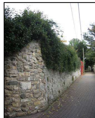
Plate 39. - Chare House wall.
