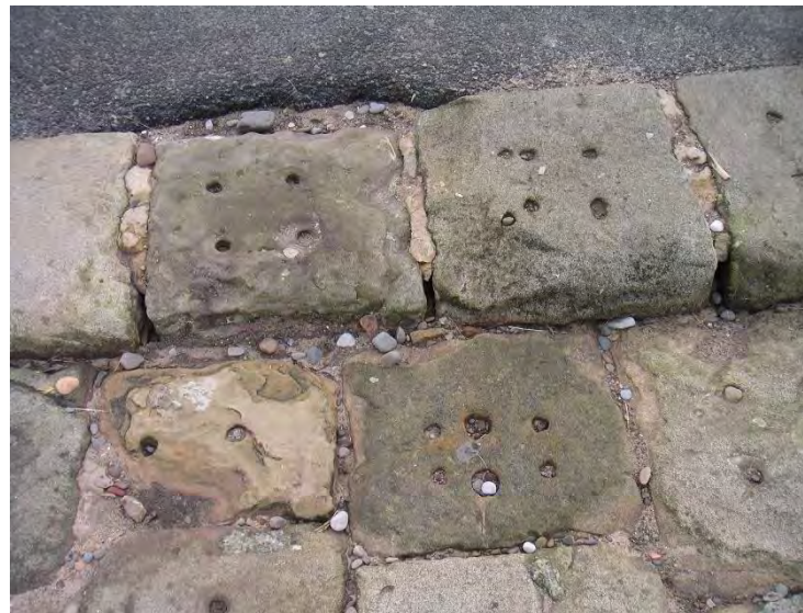
Figure 16: Granite sleeper blocks from the Stockton & Darlington Railway, re-used to construct a double-slipway at Saltburn, Redcar & Cleveland.
