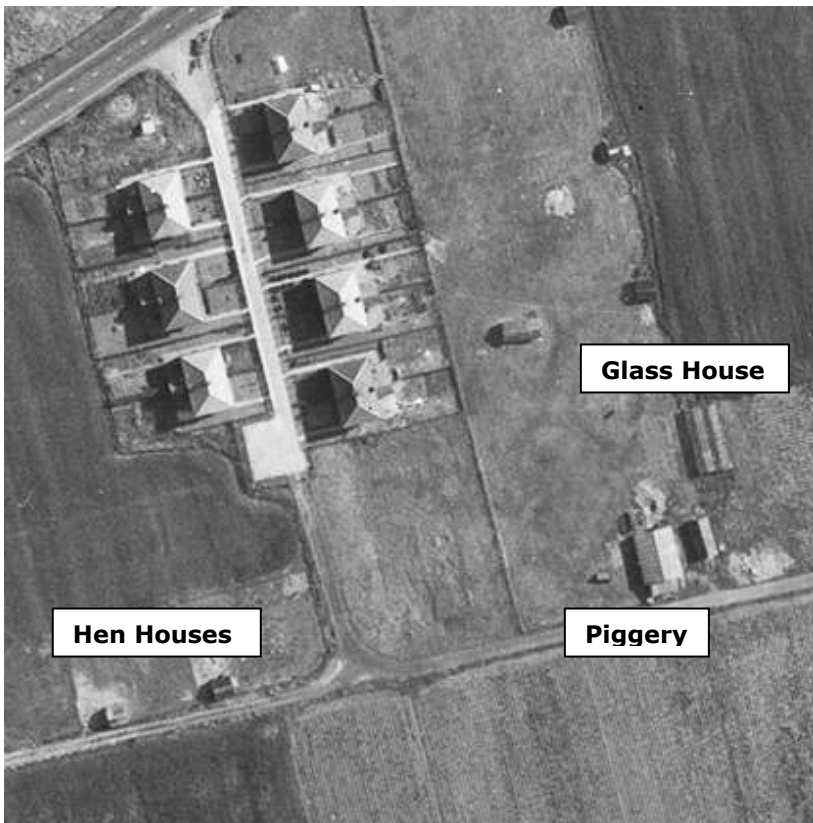
Figure 2: Nine Acres, detail of Buildings of Smallholdings (RAF/58/B/59/5559, English Heritage (NMR) RAF Photography)
