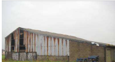
Fig 26: Burns Close, Dairy, Structure B/BCP/1
