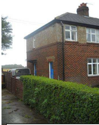
Fig 52: No 31 The Fens, front view
