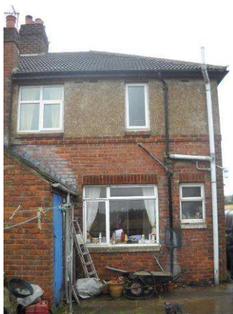
Fig 4: Rear View, No 31 The Fens
