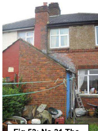
Fig 53: No 31 The Fens, rear view
