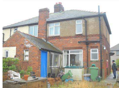
Fig 20: Rear of No 11 Burns Close
