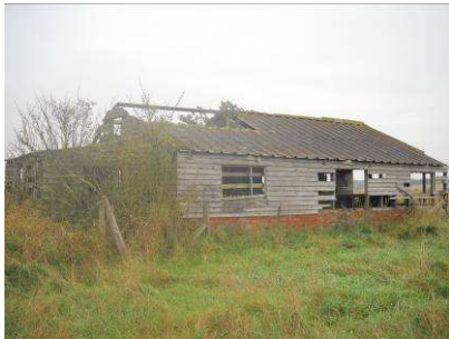
Fig 32: Burns Close, Piggery, Structure B/BCP/5
