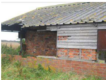
Fig 30: Burns Close, Piggery, Structure B/BCP/3
