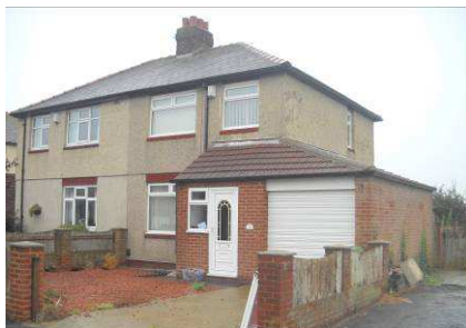
Fig 23: No 14 Burns Close The front and side elevations retain their original window openings but with replacement windows. The entrance to the property is now to the front through the extension. .....
