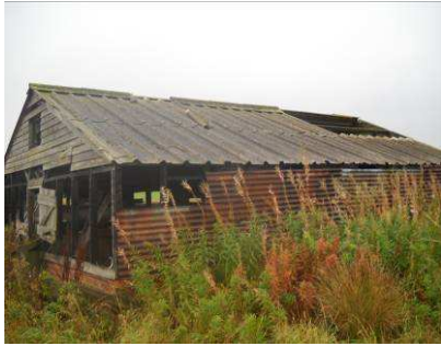
Fig 31: Burns Close, Piggery, Structure B/BCP/4
