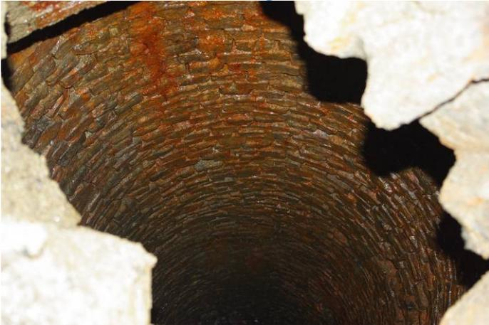
Engineers carrying out environmental improvements on Stockton High Street were surprised to discover a deep well-shaft hidden inches beneath the pavement. The well still held water and was lined with hand-made bricks suggesting it was later 18<sup>th</sup> or early 19<sup>th</sup> century in date.
